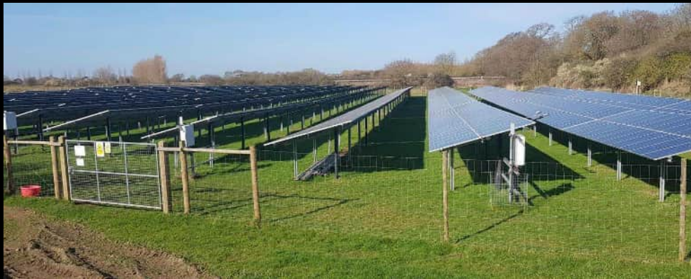
Modules mounted, finished array
